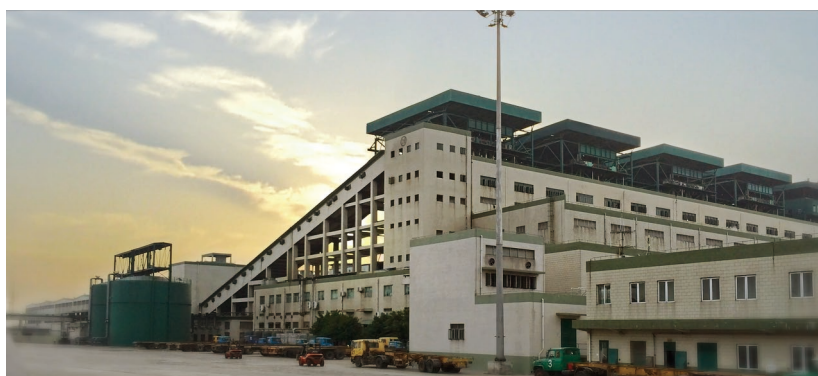
Boilers of Guangdong Lee & Man 廣東理文鍋爐
